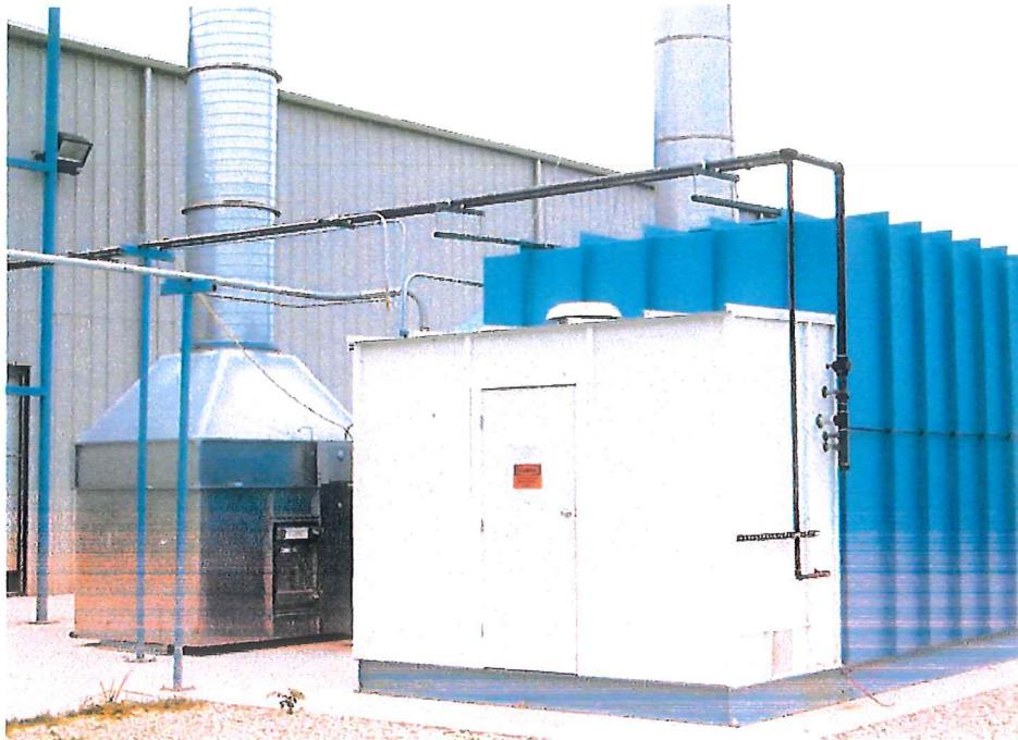
**Spectrum Metal Finishing has completed installation of their Tellkamp Systems Roxidizer® RTO volatile organic compound (VOC) abatement system. The state of the art abatement system captures 98.7% of the emissions from the liquid paint line and sends them to the Roxidizer® regenerative thermal oxidizer for destruction.**
